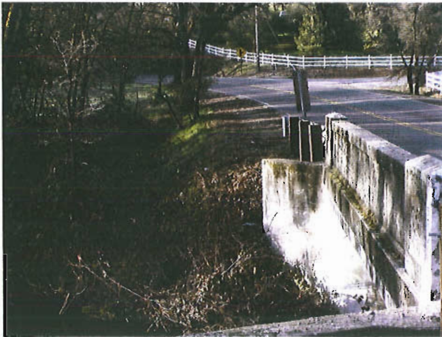
Looking South toward southeast quadrant of existing structure
