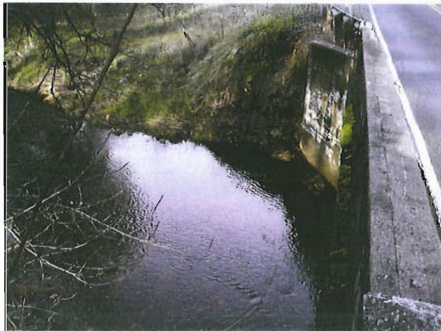
Looking Downstream (Northeast corner of exist. Bridge)
