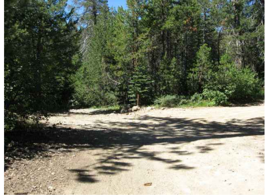
PHOTO D (Sept 2010) View of Abutment 1 location.
