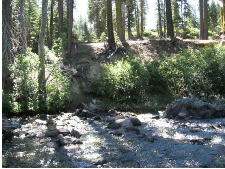
PHOTO I (Sept 2010) View of SE creek bank south of Abutment 2.
