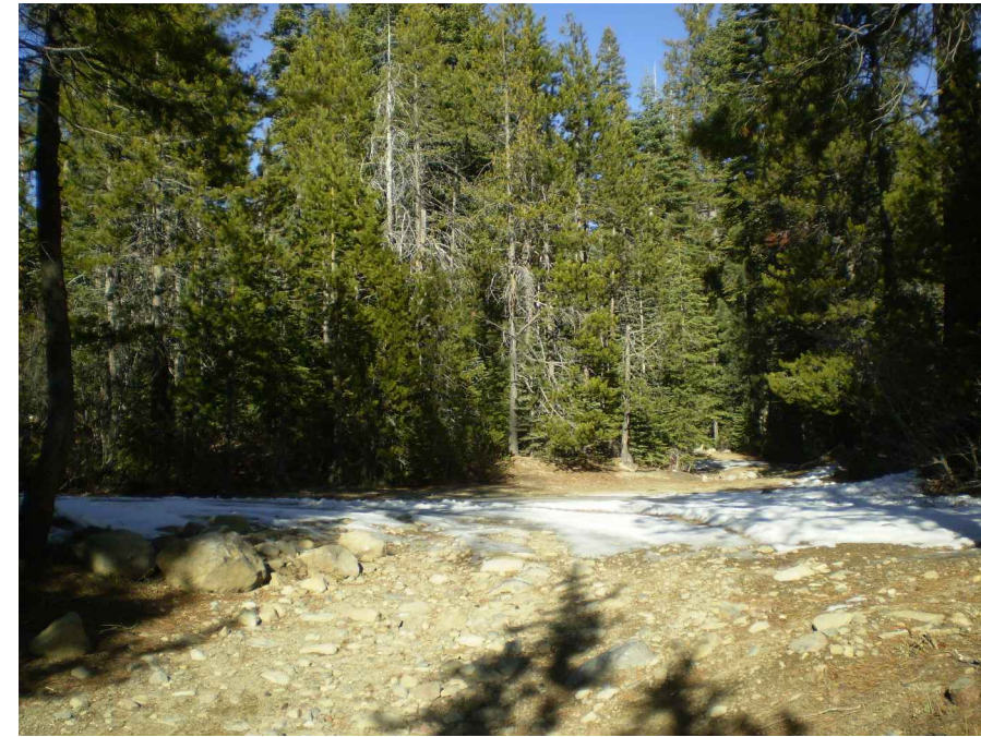
PHOTO F (Dec 2011) View of Abutment 1 location.
