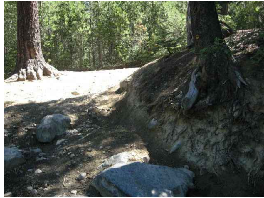
PHOTO J (Sept 2010) View of Abutment 2 location.
