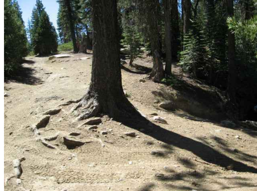
PHOTO L (Sept 2010) View of Abutment 2 location.
