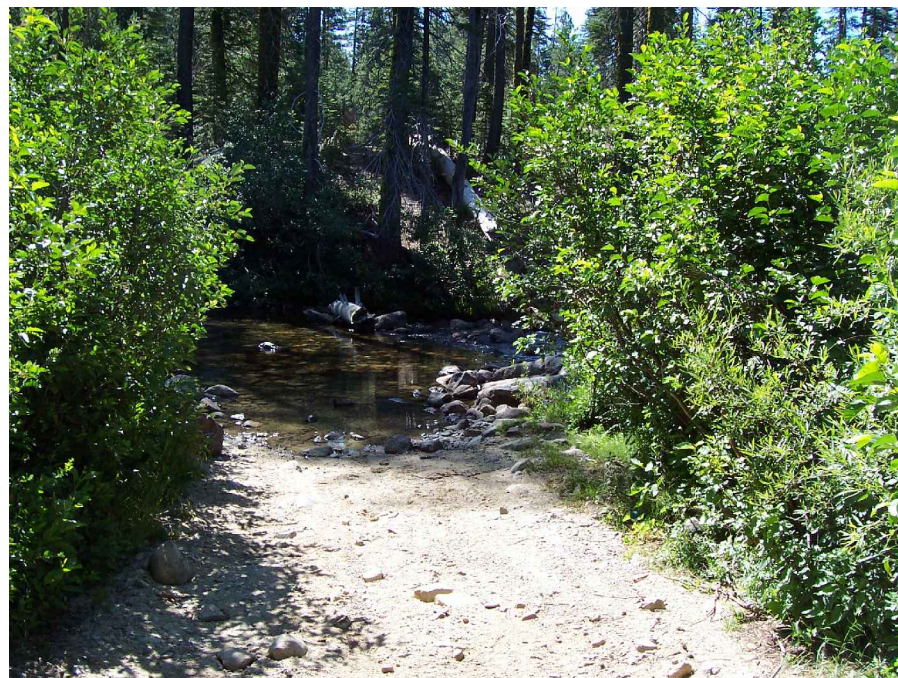
PHOTO G (Aug 2006) View of existing low water crossing on Abutment 1 side of creek.
