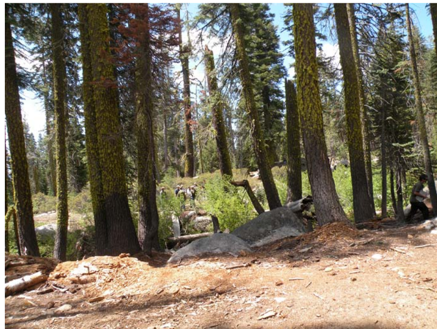
PHOTO A View of Abutment 2 location.
