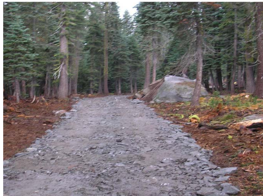
PHOTO K View along access road (14N05 to Rubicon Trail).
