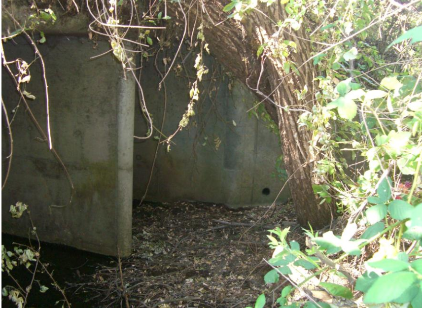
Figure 5 – Existing Entrance Conditions at the Highway 50 Buck’s Ravine Crossing
