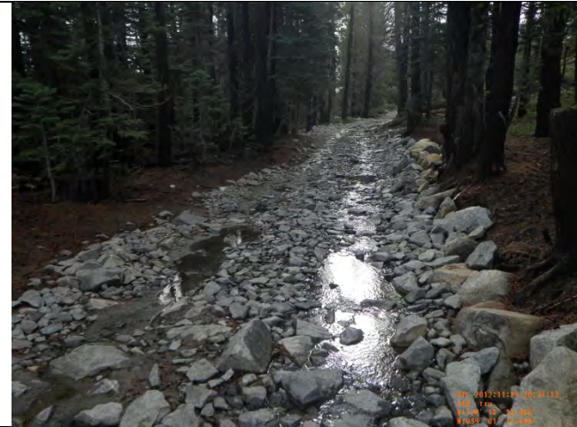
Rock Fill RT Station 104+49.21
