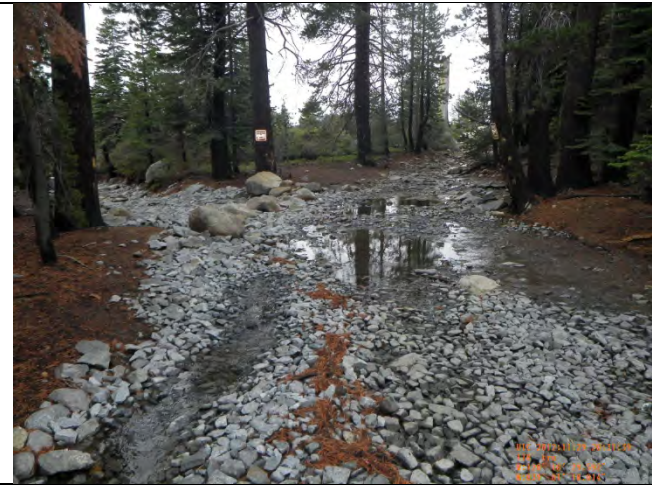
Rock Fill RT Station 99+51.63
