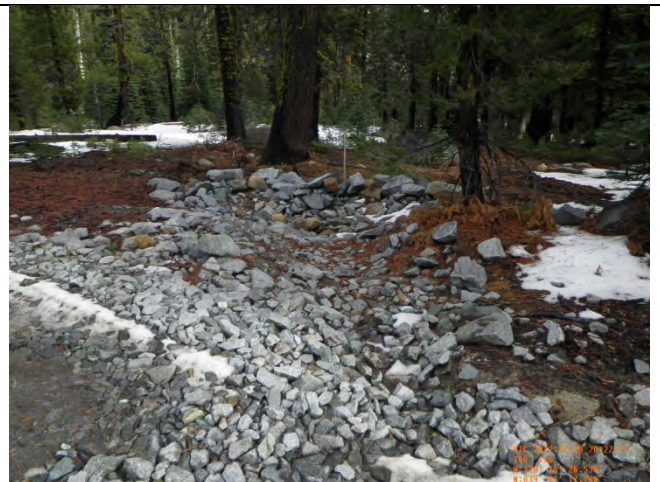
Rock Energy Dissipater RT Station 110+08.97
