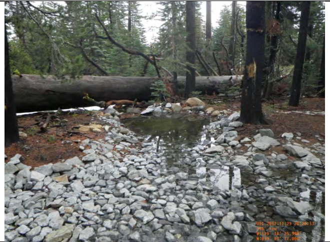
Rock Energy Dissipater RT Station 105+71.31
