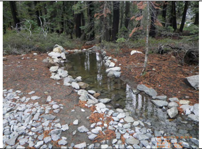
Rock Energy Dissipater RT Station 99+86+.95
