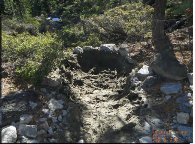
Rock Energy Dissipater RT Station 174+00 Post-Clean
