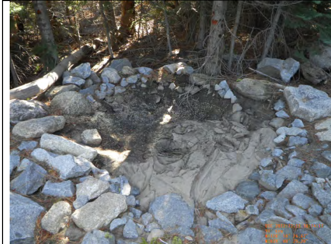
Rock Energy Dissipater LL Station 148+75.49 LT Pre-clean
