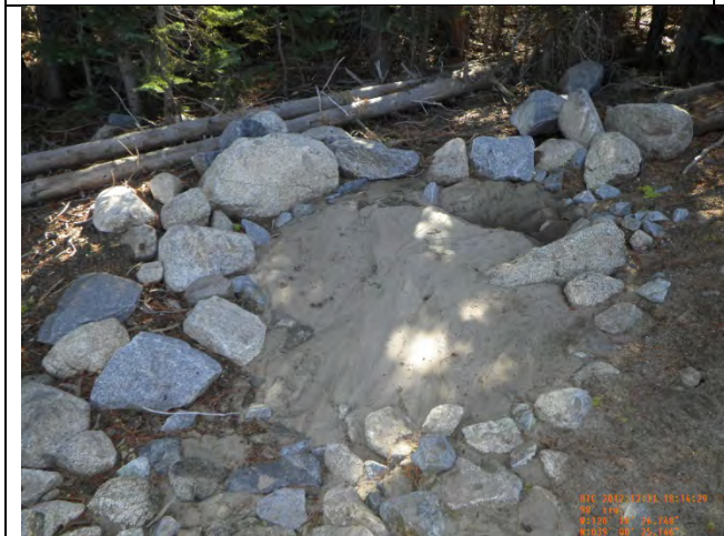
Rock Energy Dissipater LL Station 148+75.49 RT Pre-Clean
