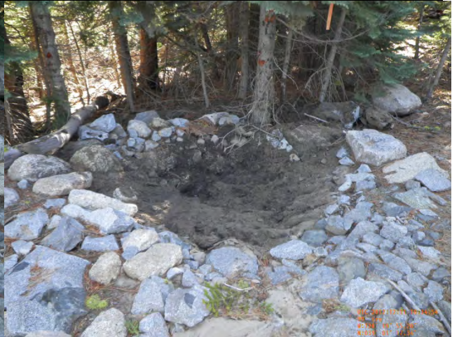
Rock Energy Dissipater LL Station 148+75.49 LT Post-Clean
