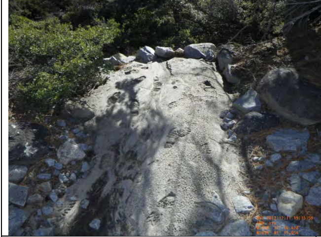
Rock Energy Dissipater RT Station 174+00 Pre-Clean
