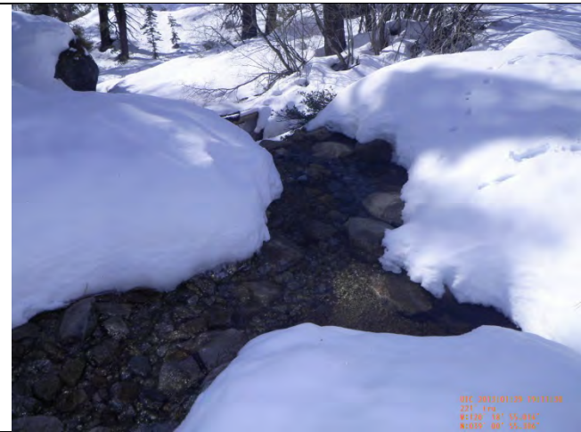
Post Pile RT Station 75+00
