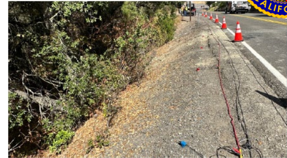
Photo 1: Segment of proposed boardwalk at approximately STA 28+00, looking northeast.
