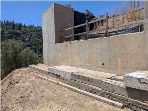
8/04/25 – Abutment 4 End Span Began Falsework Pads
