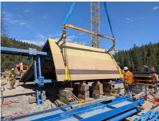
7/30/25 – Pier 3 Girder / Overhang Traveler Form Hoist
