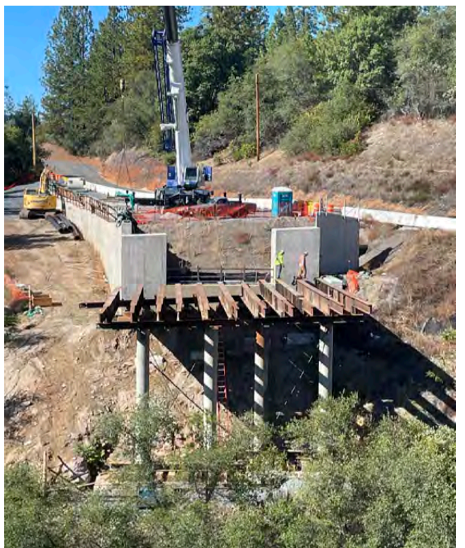
10/15/25 – Abut 4 Placed Falsework Stringers
