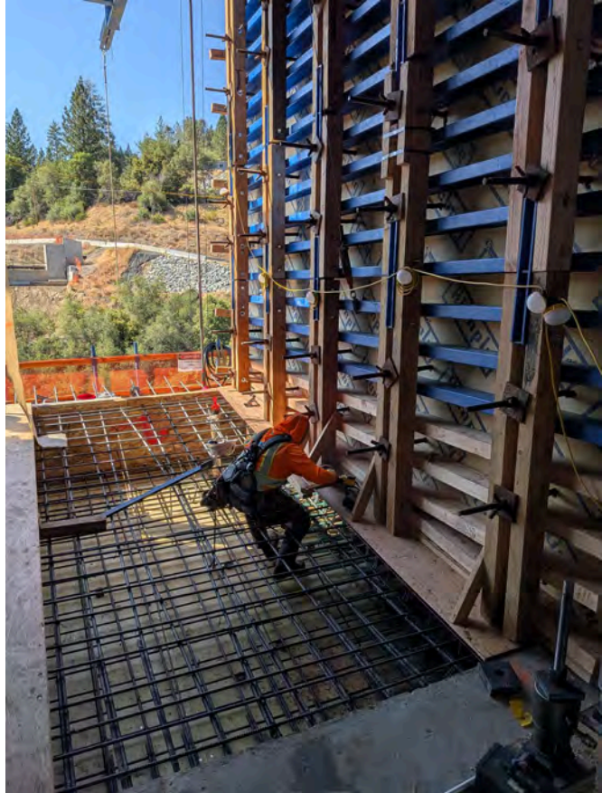
8/15/25 – P3-1E Forms Prepared for Concrete Placement
