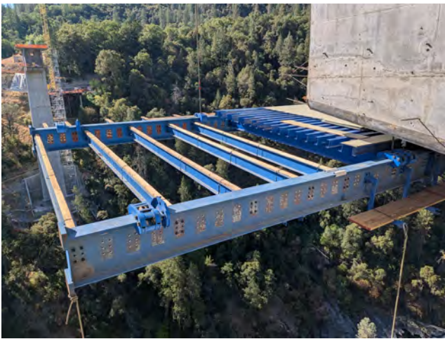
7/25/25 – Pier 3 Mainspan Bottom Platform Placed
