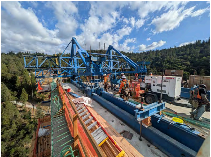
9/08/25 – Abut 4 End Span Began Falsework Posts 9/10/25 – P3-1M Launched Traveler to P3-2M
