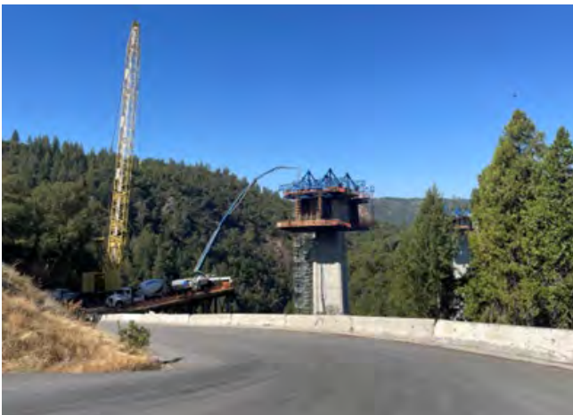
9/27/25 – P2-1E Concrete Placed
