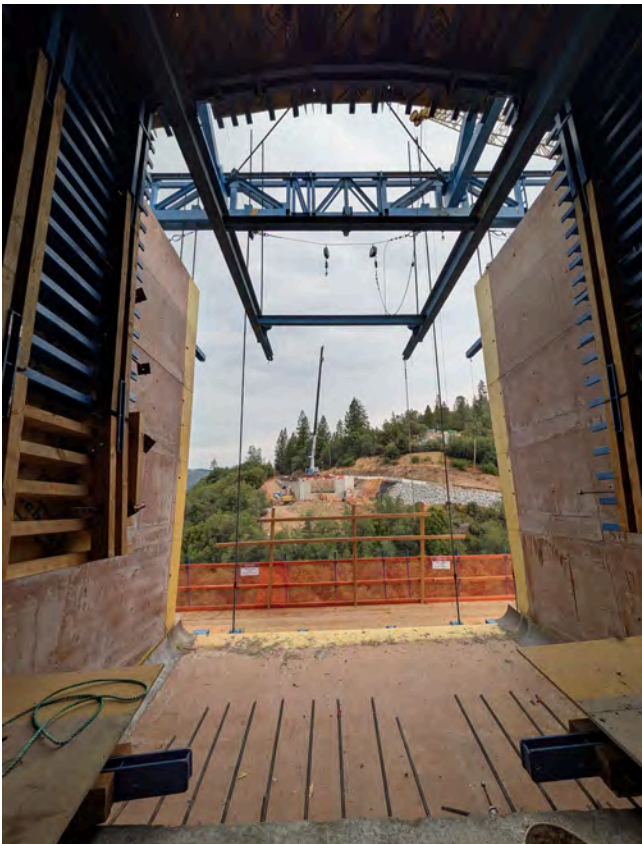
9/02/25 – P3-2E Launched & Ready for Rebar
