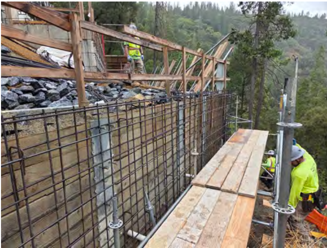
7/01/25 – Pier 2 Installed Shotcrete Rebar & Scaffolding
