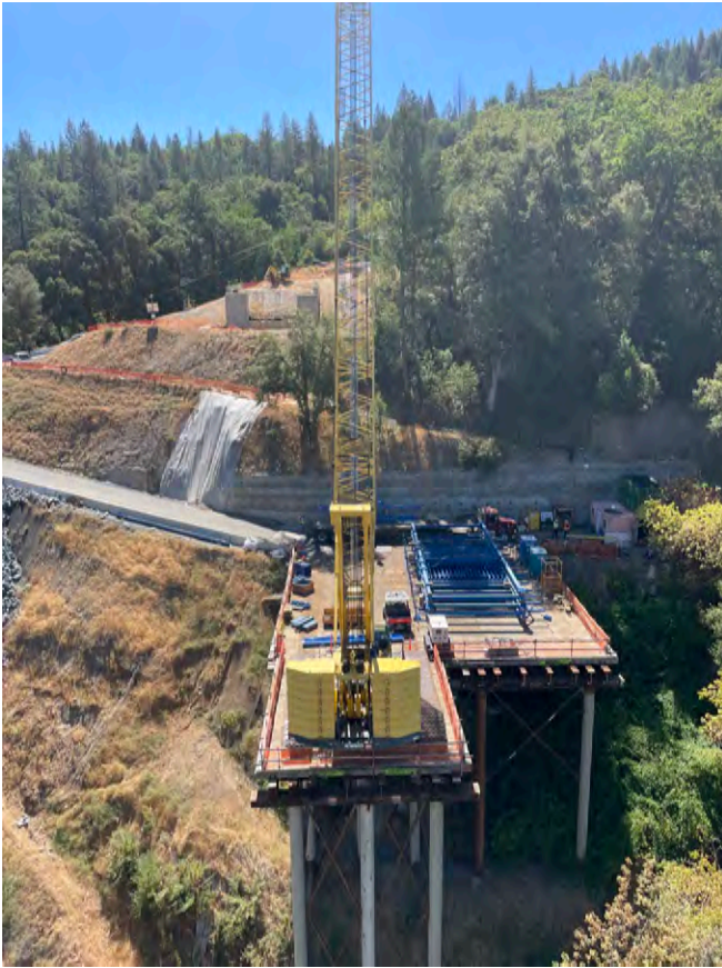
8/08/25 – Pier2 MFT Bottom Platform Constructed & Staged
