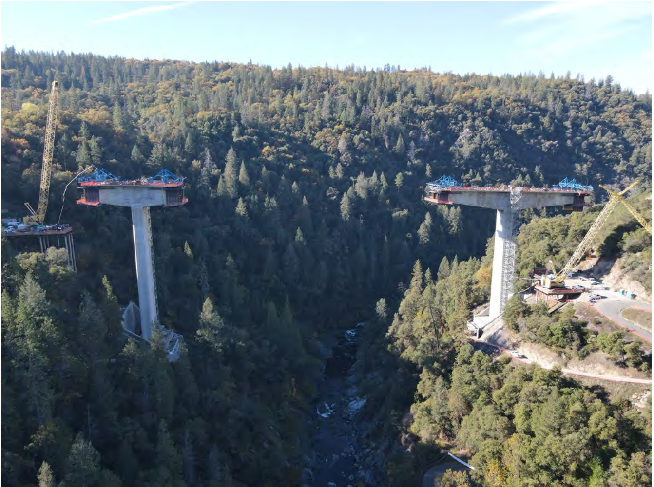
11/06/25 – Pier 2 & 3 Pier Tables & Modular Form Travelers (MFTs) & Segments Casting Progress Looking West
