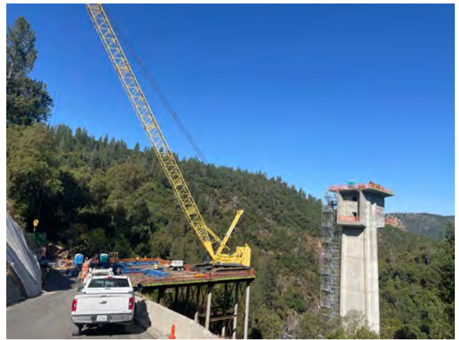
7/25/25 – Pier 2 Traveler Equipment Staged at Trestle
