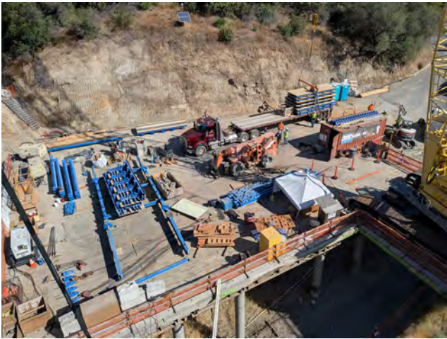
7/25/25 – Pier 3 Traveler Platforms Staging & Construction
