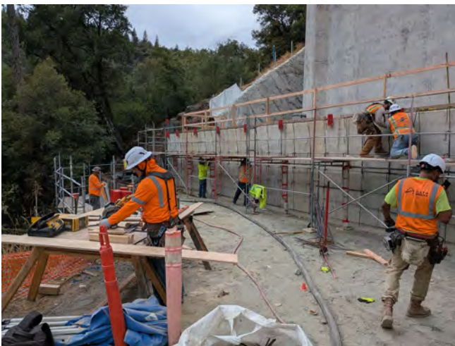
10/01/25 – Pier 3 Completed Preparation for Shotcrete
