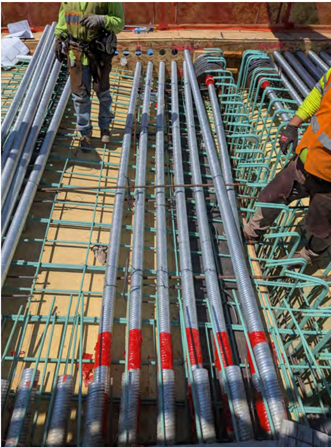
8/11/25 – Pier 3 (P3-1E) Deck Post Tensioning Ducts Installed
