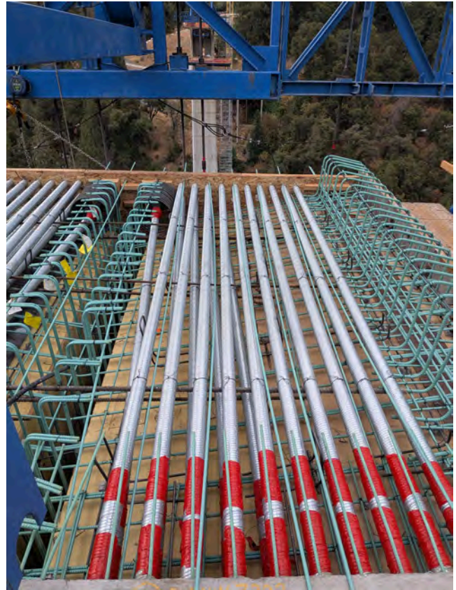
9/02/25 – P3-1M Post Tension Ducts Installed
