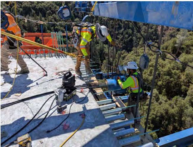
8/18/25 – P3-1E Post Tensioned Tendons
