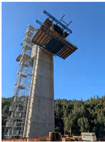
8/01/25 – Mosquito Closure Crane Maint. 8/01/25 – Pier 3 Modular Form Travelers (MFT) 8/04/25 – Placed MFT Deck Soffit
