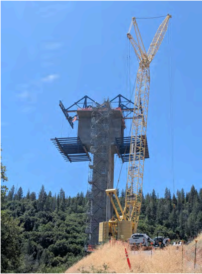
7/23/25 Pier 3 Pier Table & Began Assembly of MFTs
