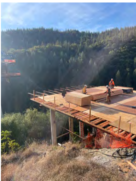
10/24/25 – Completed Joist & Soffit
