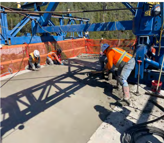
9/17/25 – P3-2E Deck Concrete Placed
