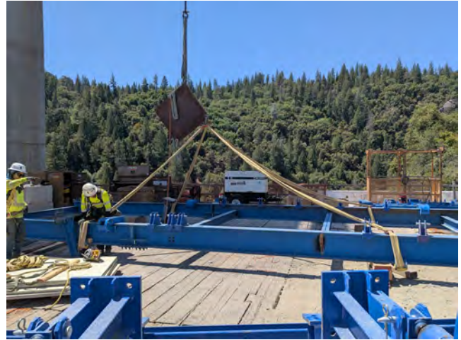
7/25/25 – Pier 3 Traveler Bottom Platform Hoist
