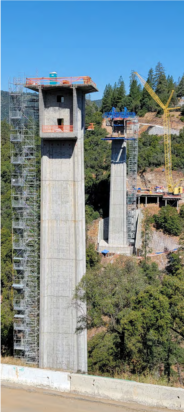
7/25/25 – Pier 2 & 3 Pier Tables & Travelers Progress
