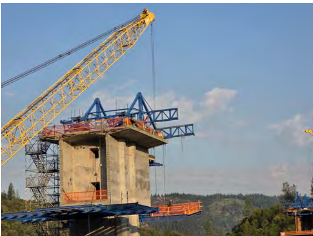
9/03/25 – P2-1E & P2-1M MFT Bottom Platforms Installed
