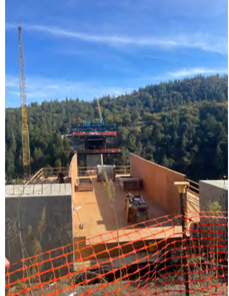
10/30/25 – Exterior Girder Forms Placed
