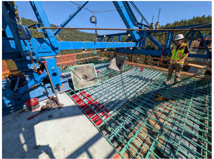
9/22/25 – P3-2M Prepared for Concrete Placement
