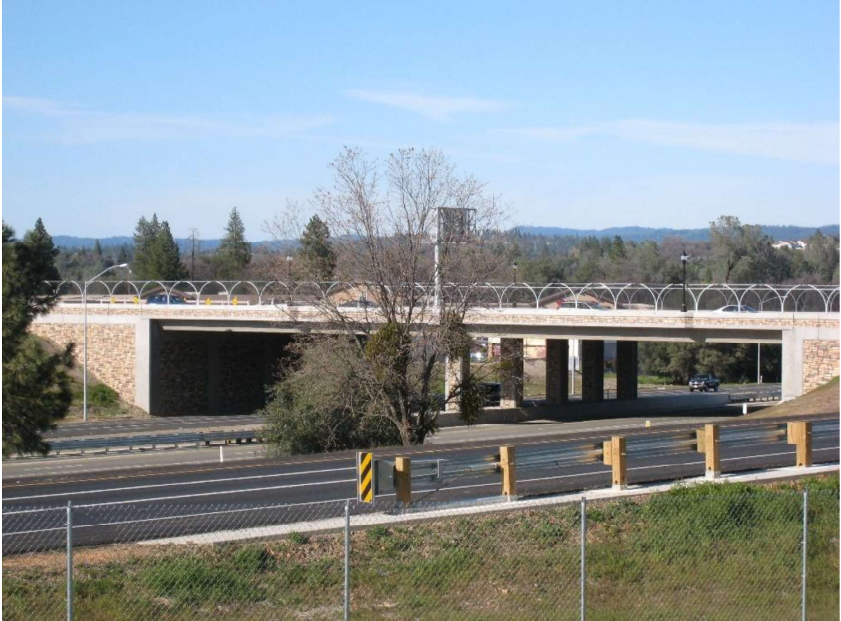
Figure 11. Example of Similar Bridge Treatment, Photo of Existing Missouri Flat Interchange
