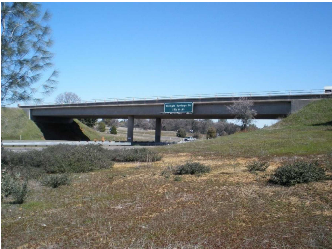
Figure 10. Existing Ponderosa Overcrossing
