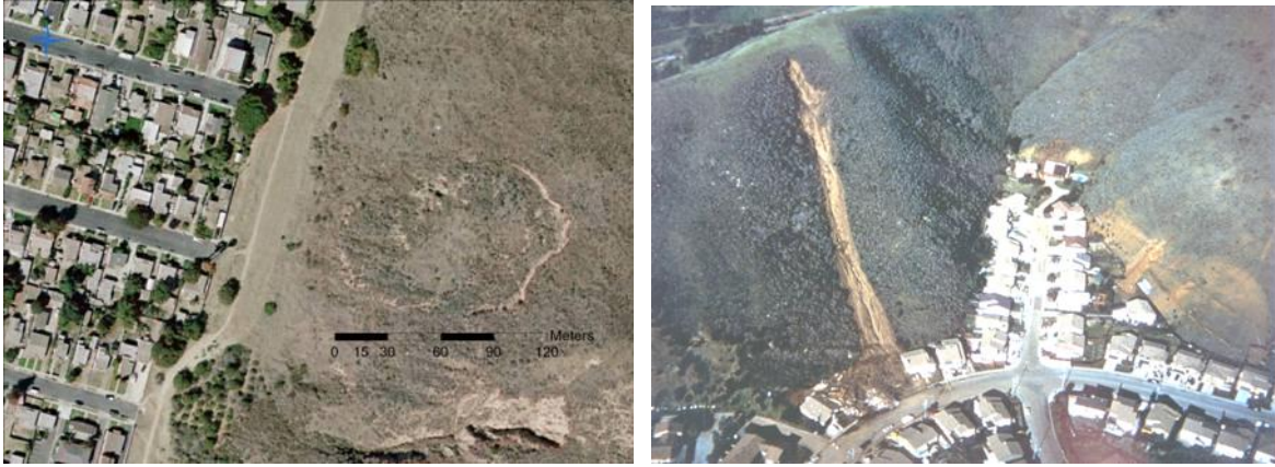
Figure 16. Deep-seated landslide in Ventura Calif., January 2005 (left, photo credit: J. Stock, USGS), and 1982 debris flow in Pacifica, Calif., that killed 3 (right, photo courtesy of Woodward Clyde Consultants).
