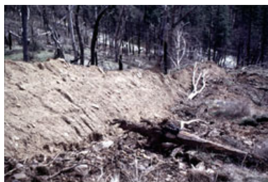
Photo 3: Lateral scarp formed by recent movement at the edge of the monitored Cleveland Corral landslide. Sliding ground is to the right of the bare soil exposed in the scarp. Highway 50 is visible (gray, upper center) below the slide. USGS Photo by Mark Reid, USGS/Menlo Park
