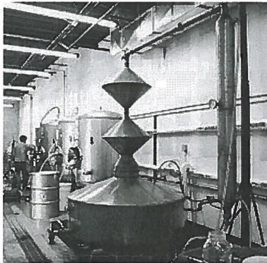
A Double Diamond pot still used by Downslope Distilling of Centennial, Colorado.
