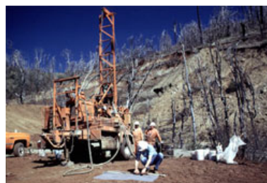
Photo 6: Caltrans drill rig installing subsurface extensometers (to measure landslide movement) and pore-water pressure sensors (to measure ground-water conditions) in the Mill Creek landslide. USGS Photo by Mark Reid, USGS/Menlo Park
