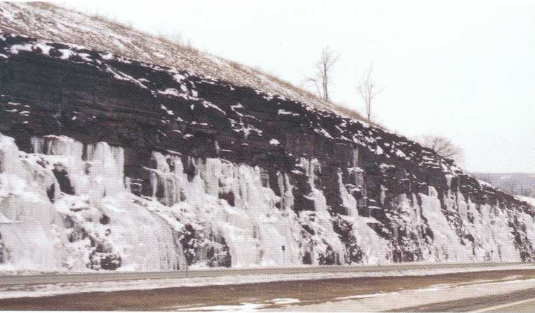
Ground water, emerging from bedding planes, has created spectacular frozen waterfalls along a road cut.
