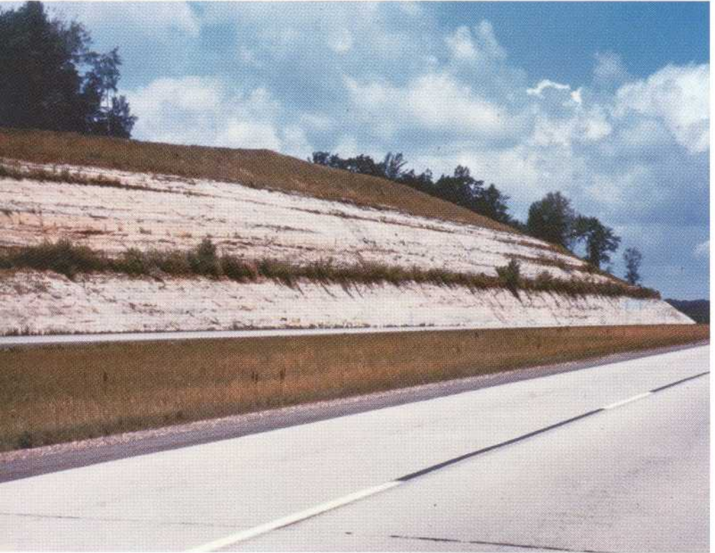
Road cuts reveal fractures, joints, and bedding planes.
