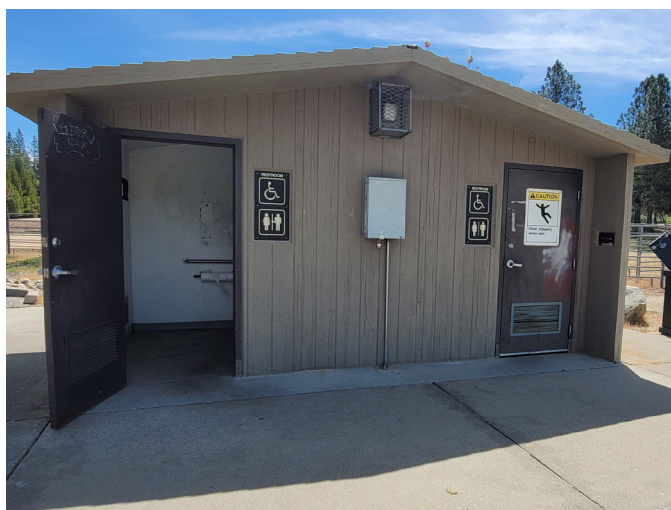
Restroom maintenance at Pioneer Park.
