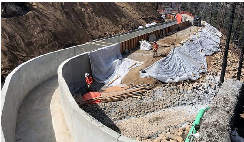
The Caldor Wildfire burned through EID’s Flume 4, 5, 6, and 30 in August 2021. Reconstruction of these flumes began in September 2021 and are now complete.
