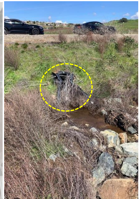
Culvert “D” in very bad shape and about 3 feet in diameter.
