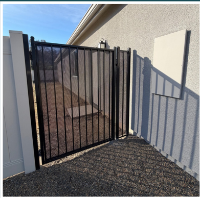
Noncombustible gate within 5 feet helps prevent fire from spreading to the structure
