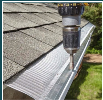
Gutter guards keep debris from accumulating near roof edge
