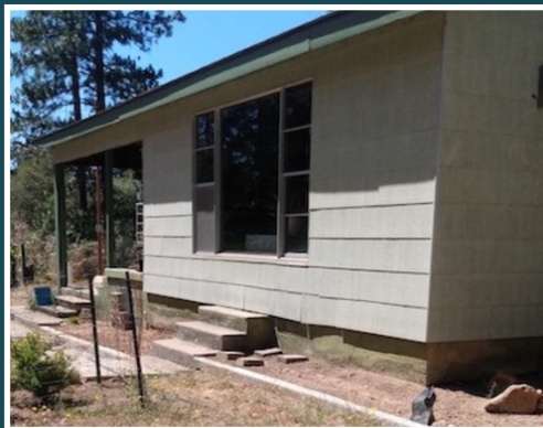
6 inch noncombustible base of exterior walls helps prevent flames or embers from igniting the structure
