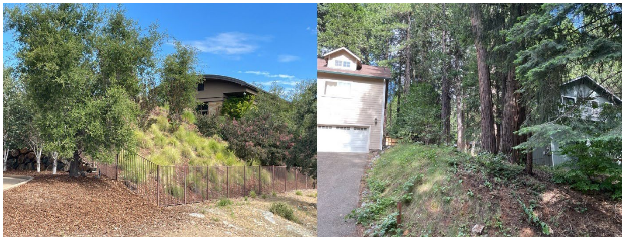
Figure 74. Many structures around El Dorado County were observed to have vegetation around the structure, including under eaves and roof overhangs, as well as between neighboring structures.
