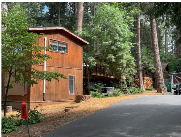
Figure 70. El Dorado County home with combustible wood siding and with stacked firewood in close proximity to the structure
