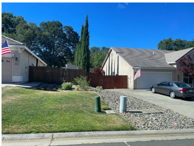
Figure 72. Two homes in El Dorado County with wood fences that are both attached to each home and near to one another. This situation can lead to fences acting like a "wick" that brings fire to structures.
