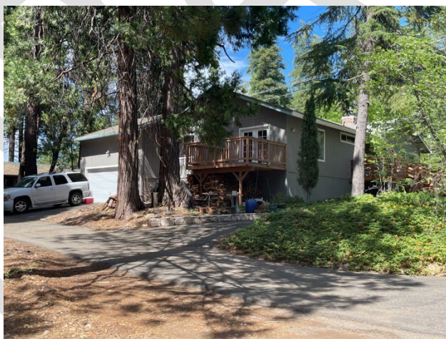
Figure 73. Wood deck attached to a home in El Dorado County, adjacent to sliding doors, and with stacked firewood stored underneath.
