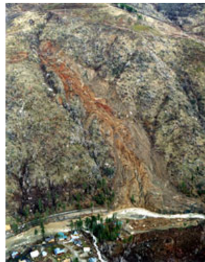
Photo 1: Aerial view of the Mill Creek landslide blocking Highway 50. Caltrans Photo courtesy of Lynn Harrison, Caltrans
