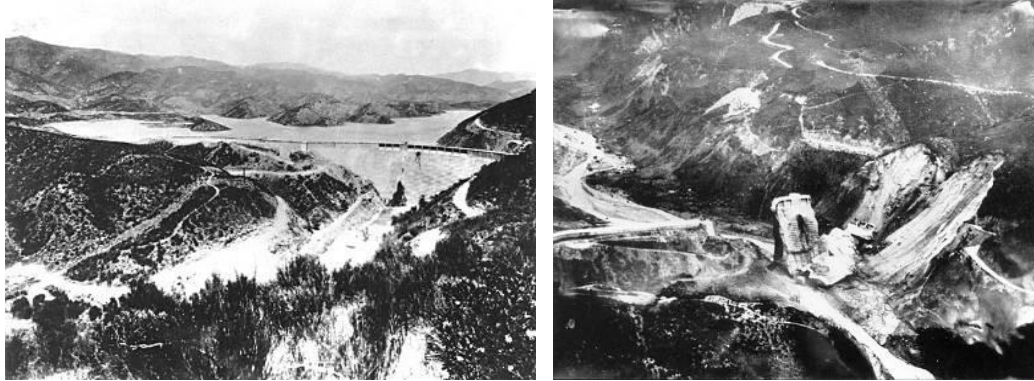
Figure 35. St. Francis Dam before (left) and after (right) collapse (both images: public domain).
